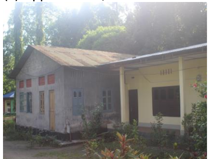
(n) West bank, Dormitory IB
